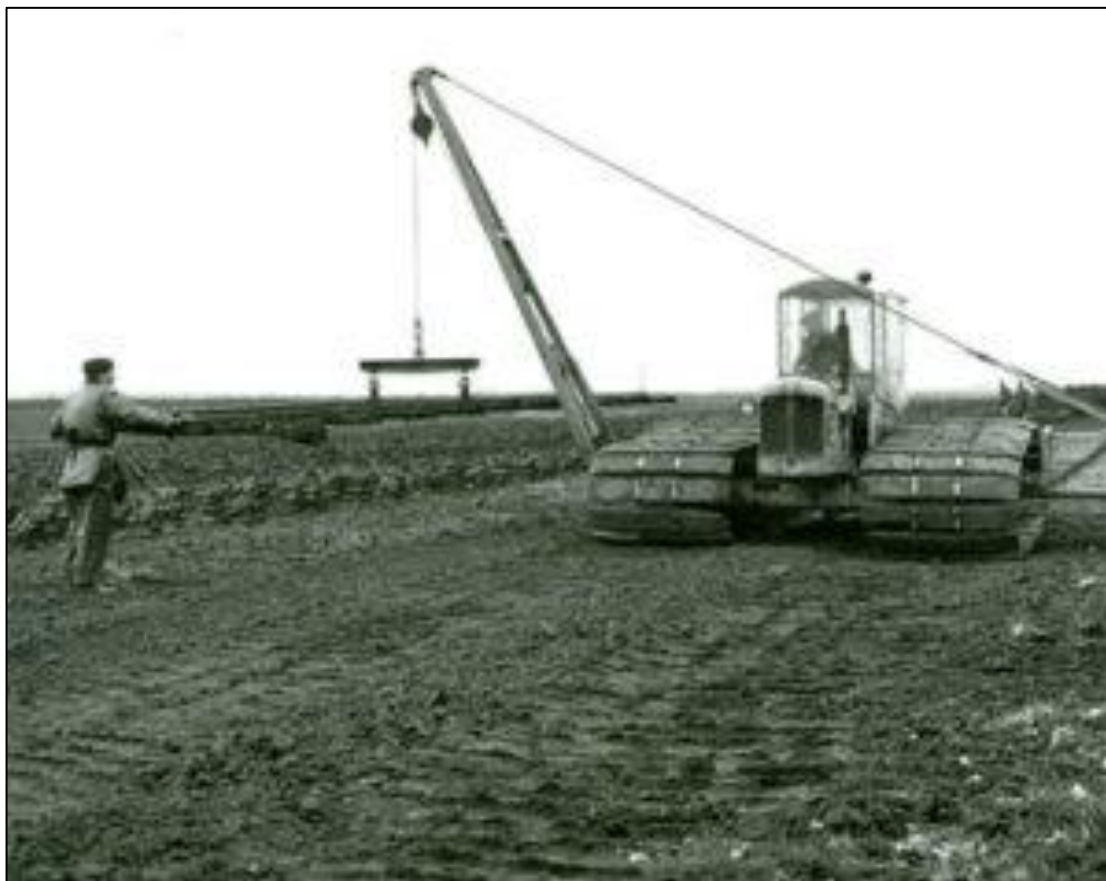
Plate 4-36 Rail Moving Attachment to lift and lay temporary railway track, along Sod Peat ricks and milled peat piles. Source: https://www.bordnaMónalivinghistory.ie/equipment-detail/rail-moving-attachment/
