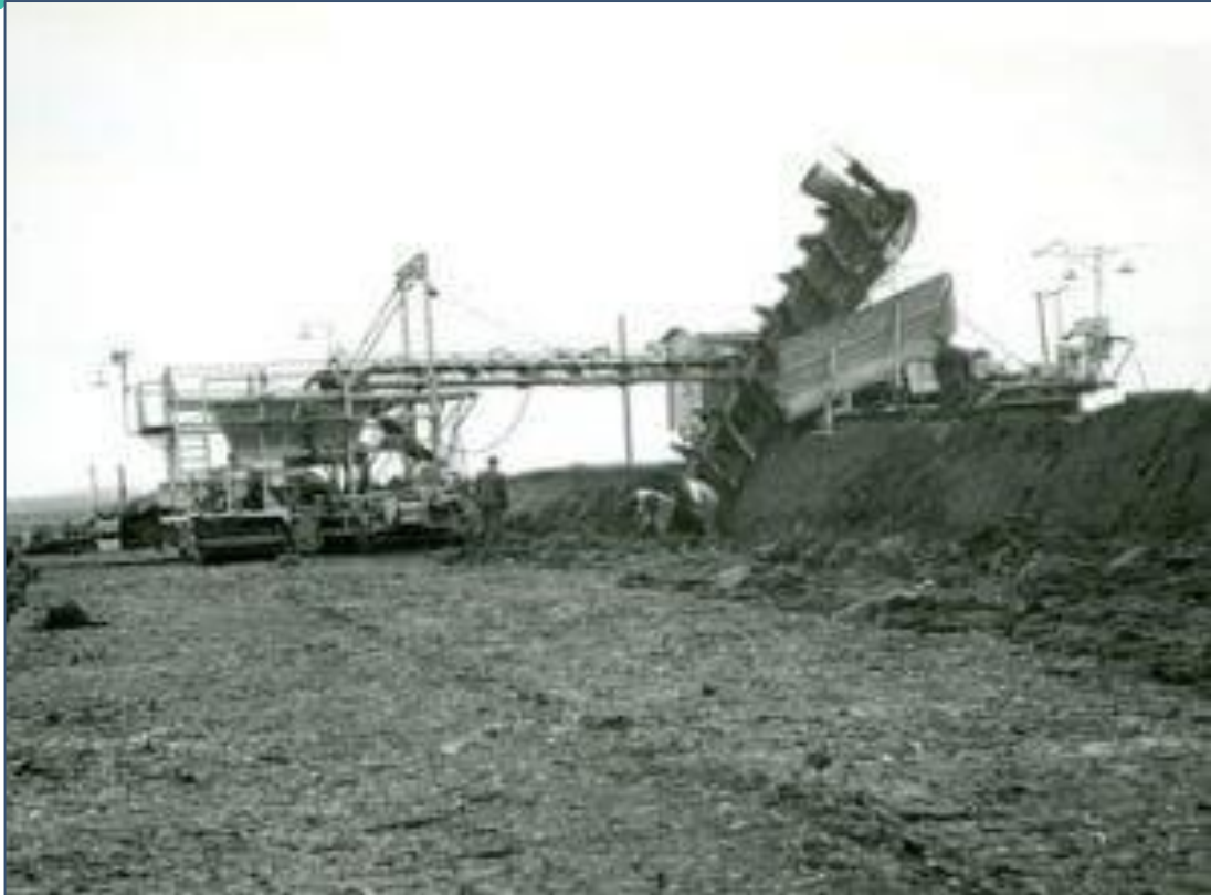
Plate 4- 22 Sod Peat Bagger/Excavator. Source: https://www.bordnaMónalivinghistory.ie/equipment-detail/sod-peat-baggerexcavator/
