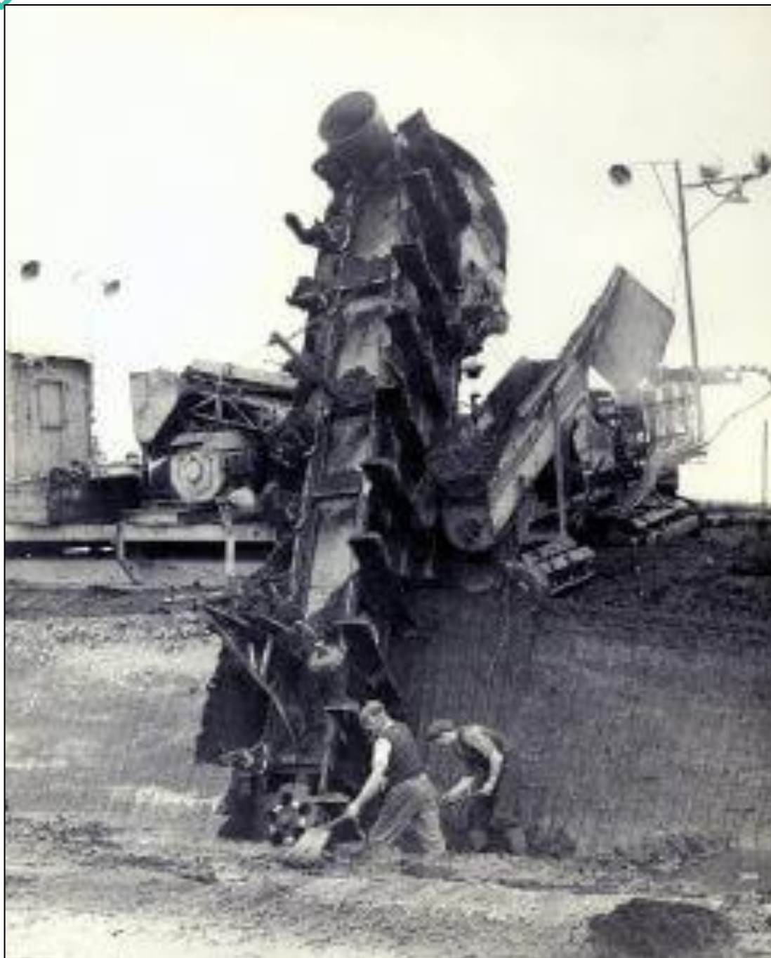
Plate 4- 21 Sod Peat Bagger/Excavator. Source: https://www.bordnaMónalivinghistory.ie/equipment-detail/sod-peat-baggerexcavator/
