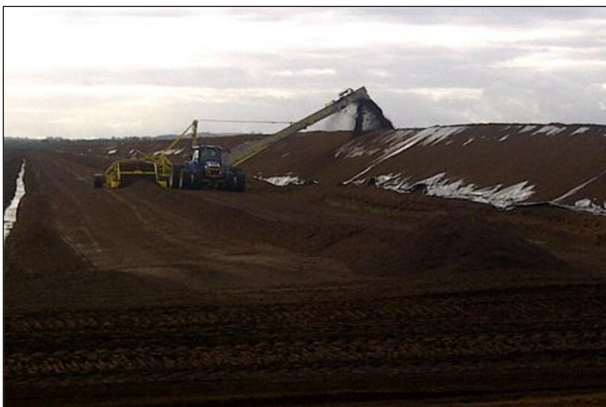
Plate 4- 16 Process of Stock Protection, showing a layer of milled peat being spread over polythene sheeting to anchor the sheeting in place (source: Bord na Móna)
